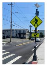
Migma Systems has developed an alternative product, Distributed Sensing Flashing Beacon (DSFB). The sensor receiver is embedded inside the housing of flasher, drawing power from solar panel or solar battery. Using solar-powered detector, it flashes only when pedestrians who are waiting at midblock curb are detected. Otherwise, it is off! The sensor response time is less than 1 second. Moreover the detector and RRFB can be installed on different poles or posts.
